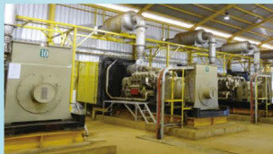
10 sets of generating units for Indonesia SILO iron ore processing plant
